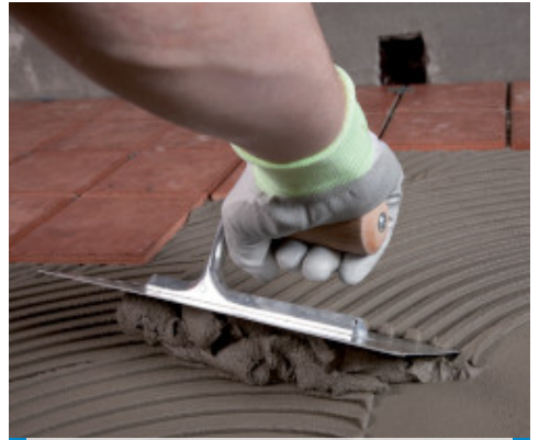
Laying Granirapid on a terrace waterproofed with Mapelastic
