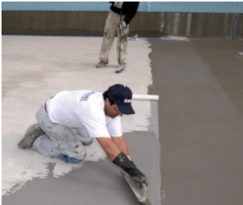
Waterproofing a swimming pool with Mapelastic
